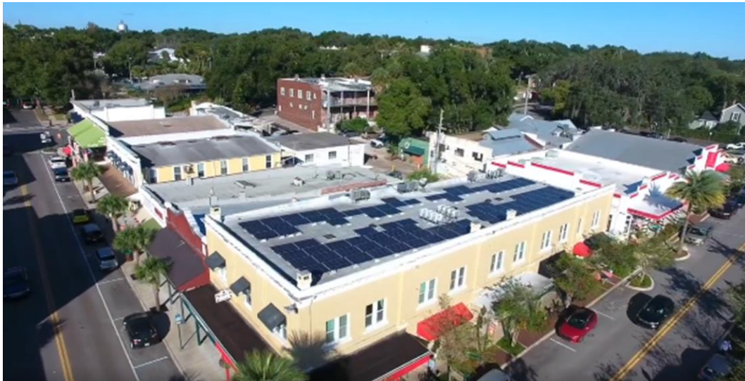
Co-op vendor Optimus Solar's commercial installation in downtown Mount Dora.
